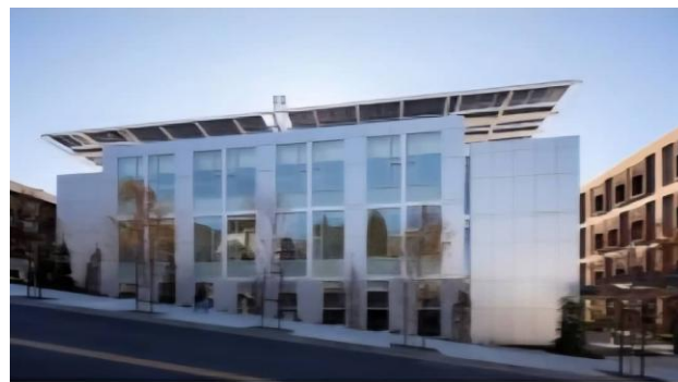
Figure 12 Illustrates the Main Ideas for achieving the Principles of Green Architecture and Its Positive Impact on Energy Conservation
